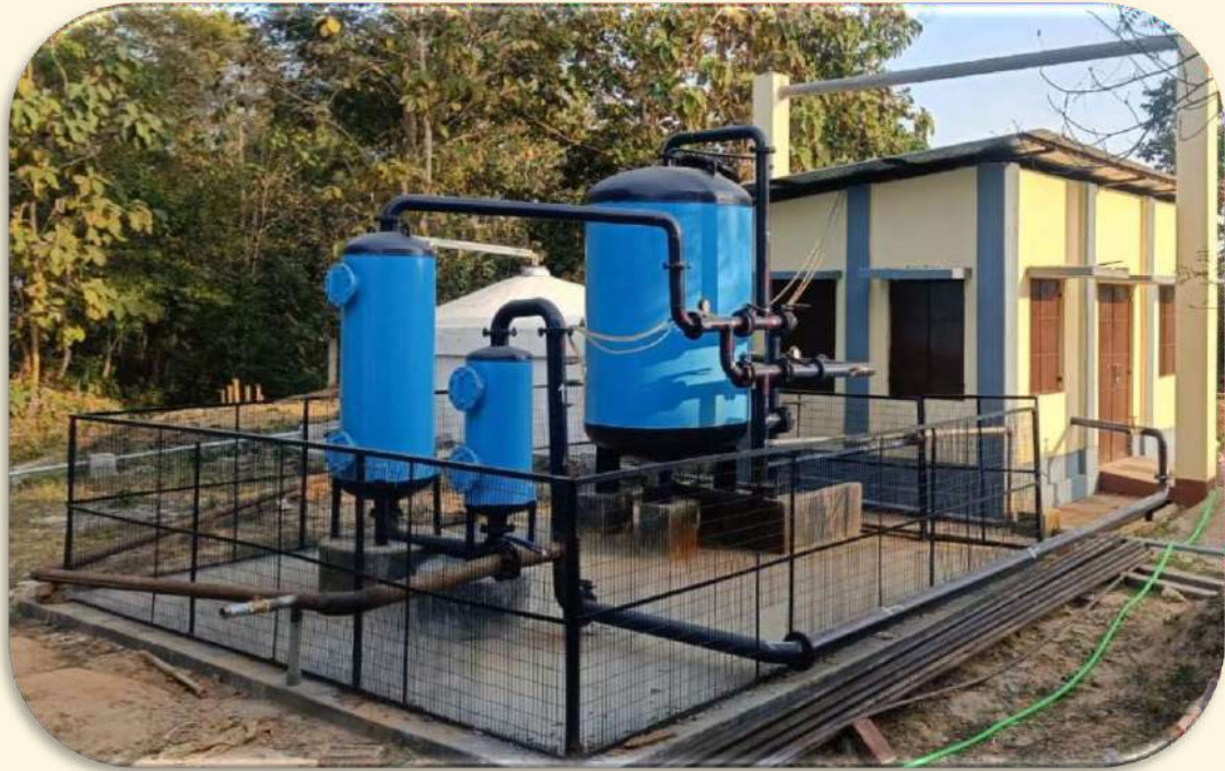
Installation of 1000 Gallon IRP at Ambassa Court Complex
